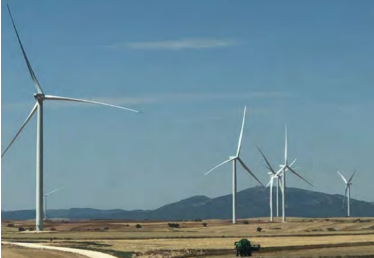
Project Goya, a 200MW Wind farm in Azuara, Aragón
