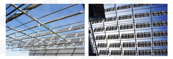
Fig. 11. PV panels installed above the outdoor hall of CEDINT-UPM building.
