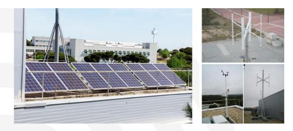
Fig. 12. Microgrid located at the rooftop of CEDINT-UPM: PV panels (left) and wind turbines (right).
