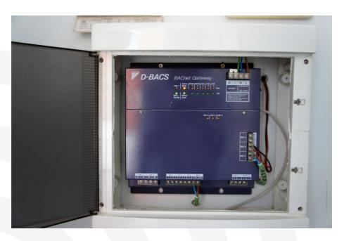
Fig. 13. HVAC control system that allows the communication with HVAC indoor units.
