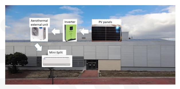
*Fig.* 18. Architecture of the PV-powered aerothermal source for HVAC of the IoT laboratory.
